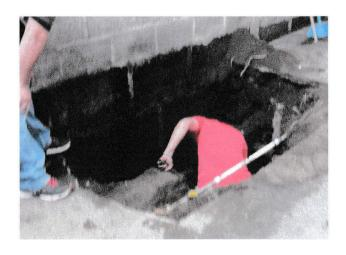
The concrete floor had to be broken up, and a lot of digging was needed to get to the pipe for repair. The damaged pipe was the neighbor's drain, which luckily did not cause a problem with the water supply for the children.
